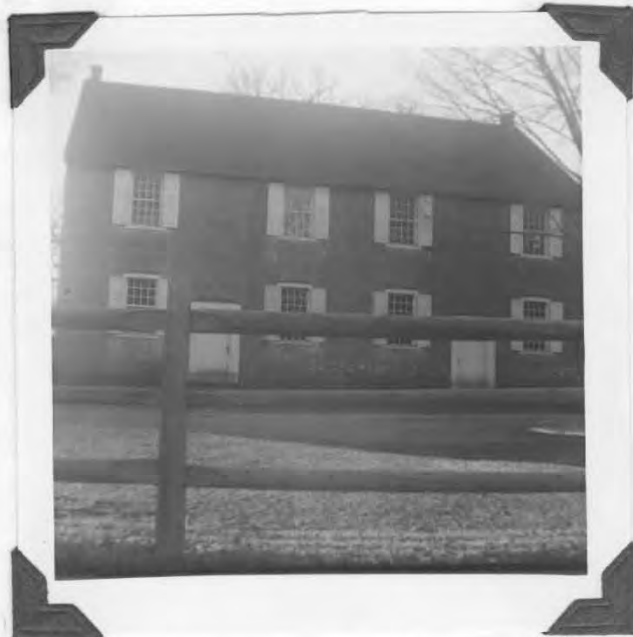
Upton's when Hoag's house burned down. A Preparative Meeting (continued on page 55)
