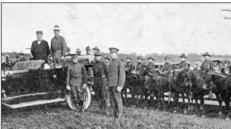
Gov. Charles Whitman and Gen. John F. O'Ryan inspect the troops at Camp Whitman in Beekman. Photo courtesy of DCHS
