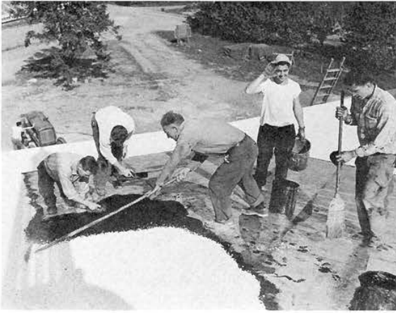
Marist Brothers working on the roof of Donnelly Hall. Photo credit: Marist College Archives
